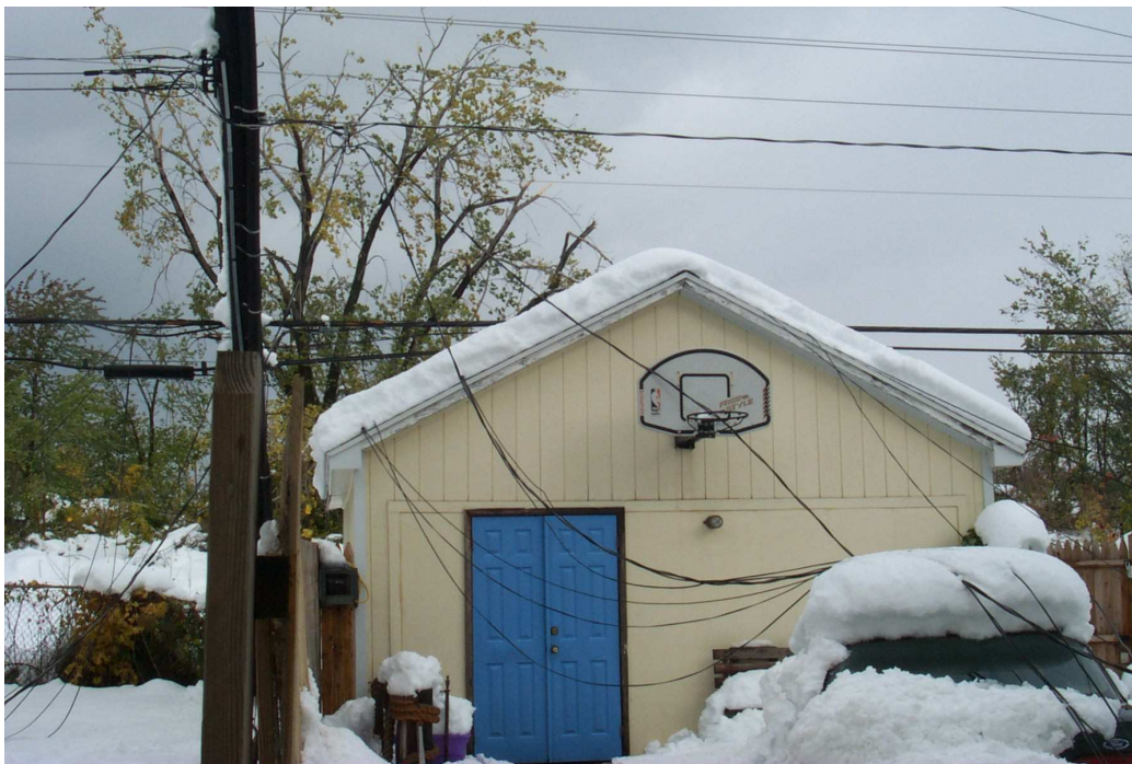
Figure 30: Another Detail of Loose Power Line
