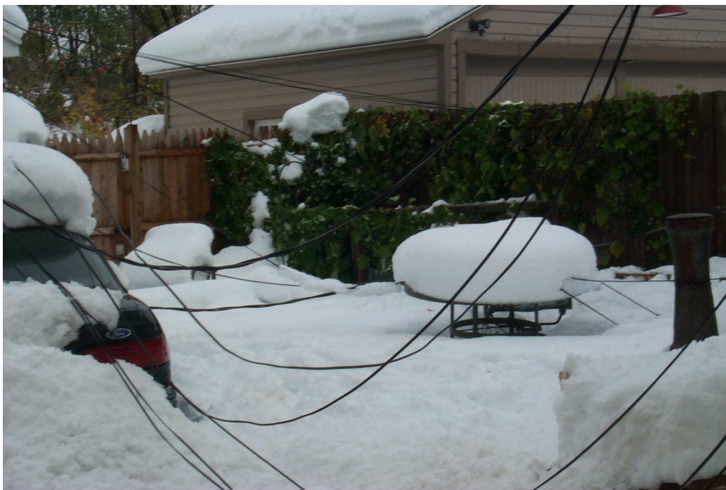
Figure 29: Detail of Loose Power Line
